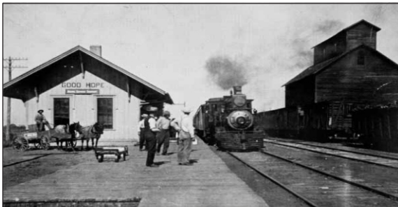
Good Hope, Illinois grain elevator
